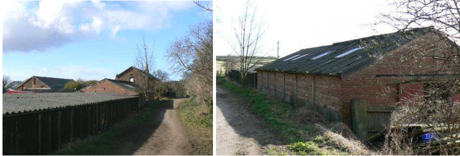
Hall Farm buildings to the south of the C19 barns
