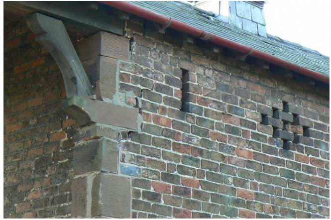
Typical vernacular brick, stone and timber detailing of Hall Farm barn,
