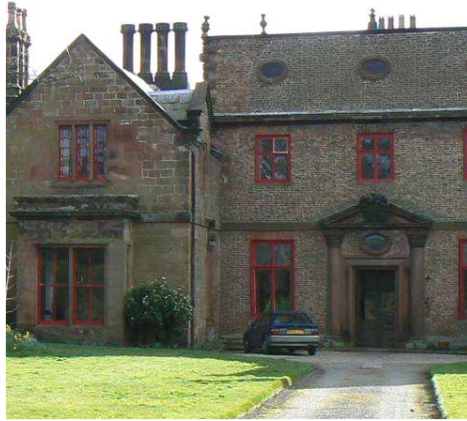
Thurstaston Hall, central section late C17 in brickwork East wing C19 in sandstone (early C17 style)
