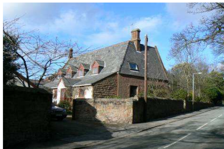
Rear extension to the old school house is not over obtrusive
